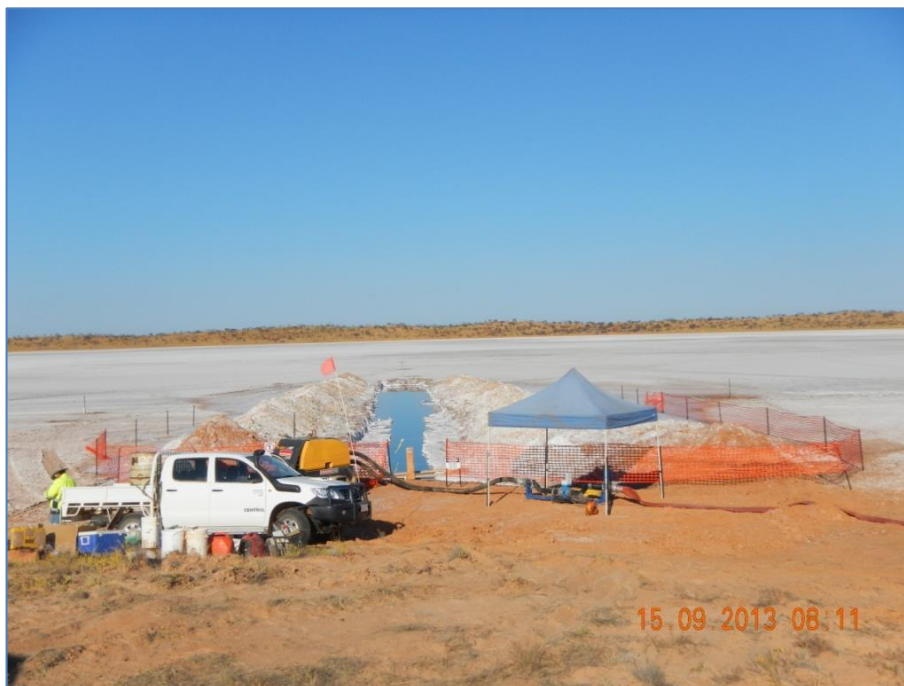
Figure 5. Pump testing at Miningere Lake.
