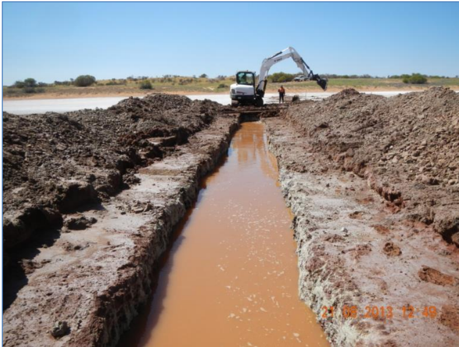
Figure 4. Miningere Trench digging in progress.
