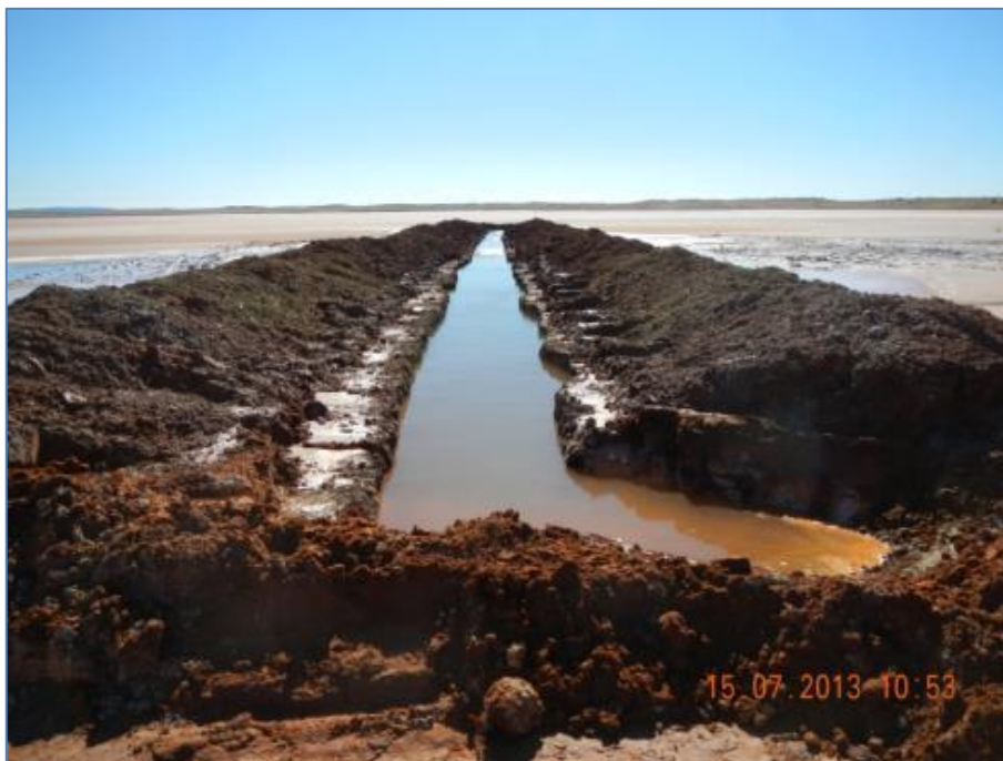
Figure 3. Newly completed trench completed at Curtin Boundary Lake, prior to fencing.
