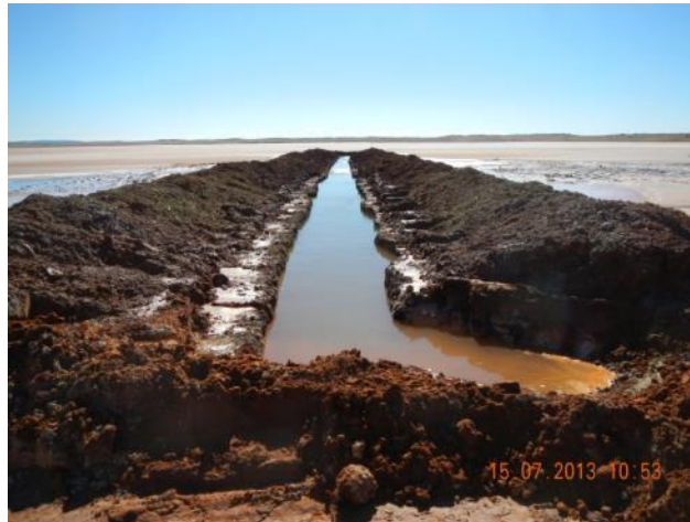
Figure 7. Trench completed at Curtin Boundary Lake
