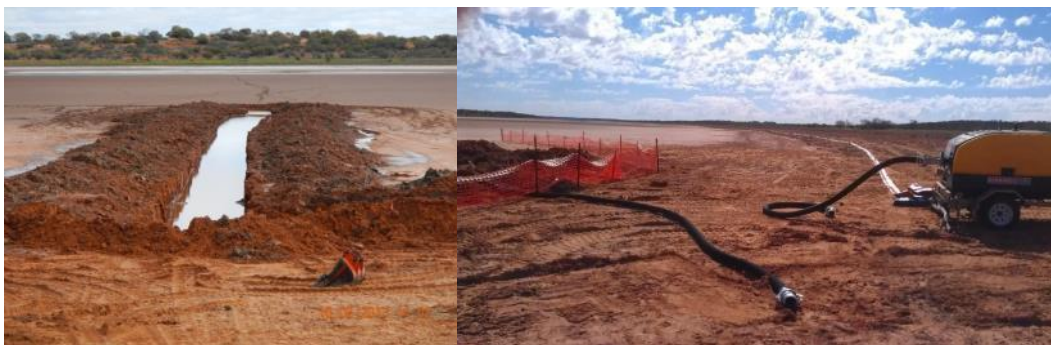
Figure 8. Trench completed and ready for pump testing at Pulcura Lake
