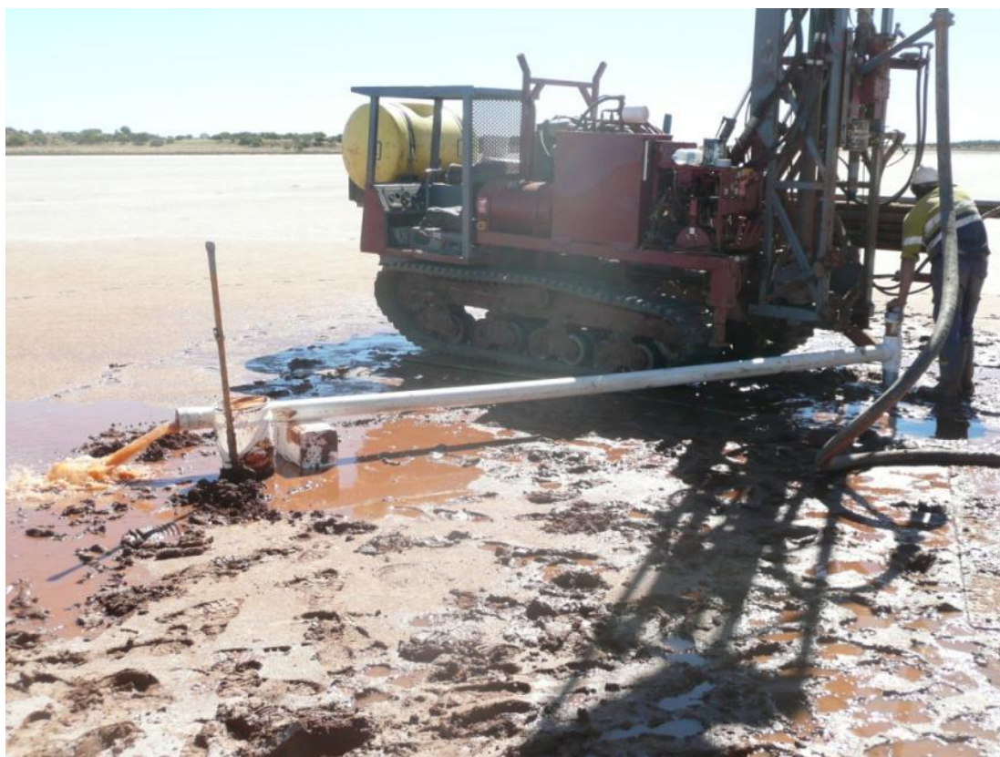
Figure 9: Flow testing a bore from 6 m depth on Pulcura Lake
