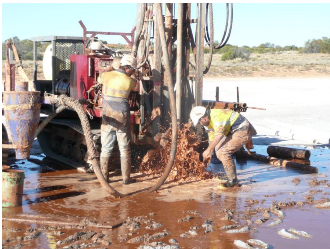
Figure 11: Brine produced during air core drilling of hole on Miningere Lake to 24 m depth
