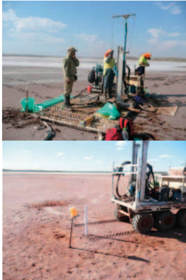
Figure 6. Sonic drilling and piezometer installation at Karinga Creek
