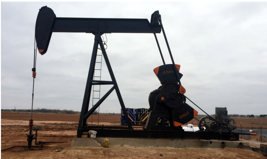
Pumping unit on the Hope Boles PU1 well
