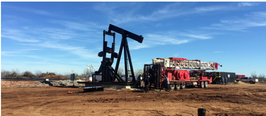
Installation of the pump unit on the McCain 189-F1 well
