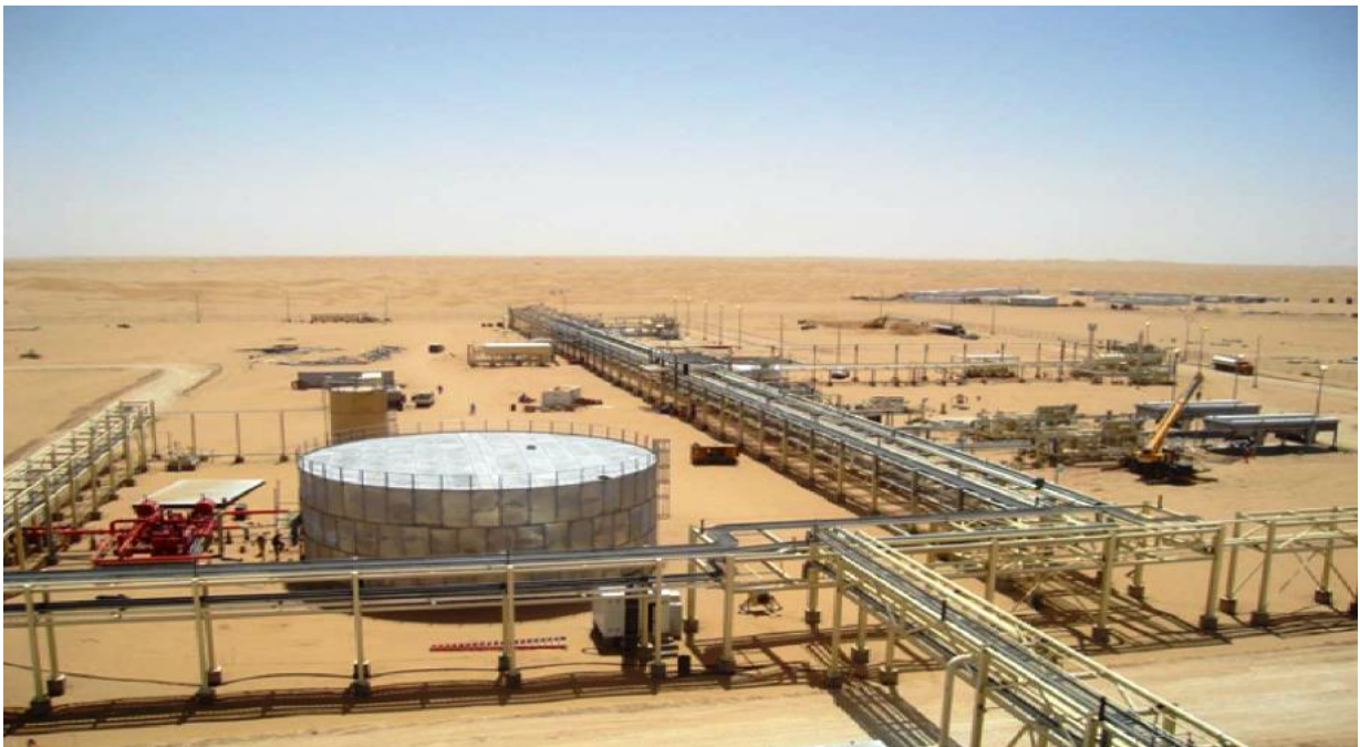
Figure 2: An Nayah Central Processing Facility with oil storage in the foreground
