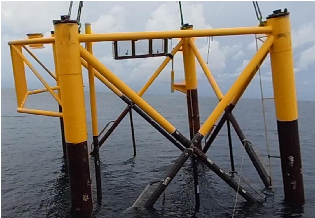
Main Pass 270 Hummer Project Jacket Installation – Jacket in the upright position
