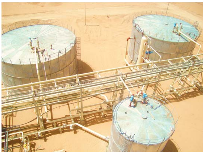
Damis (Block S-1) Production Licence – An Nagyah Oilfield production and storage facilities
