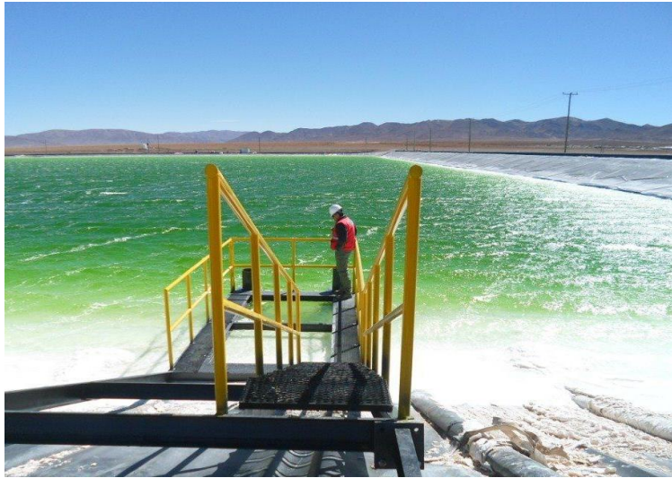
Evaporation pond post magnesium removal/lime addition
