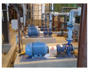
Transfer pumps in the lithium carbonate plant
