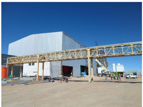
Cladding being completed on the Lithium Carbonate Plant Building after installation of major equipment
