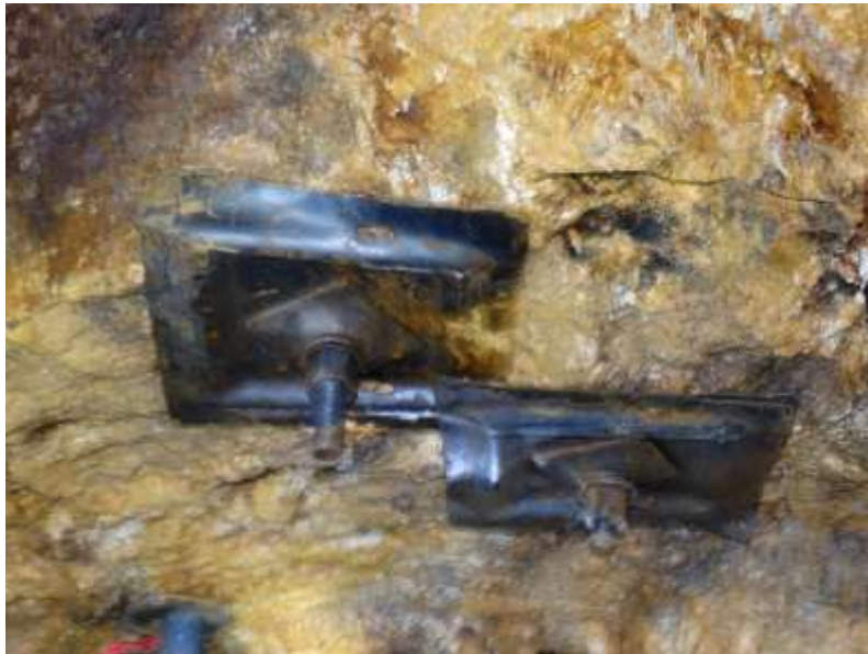
Figure 2:- Completed rockbolts no installed throughout the mine Project Schedule
