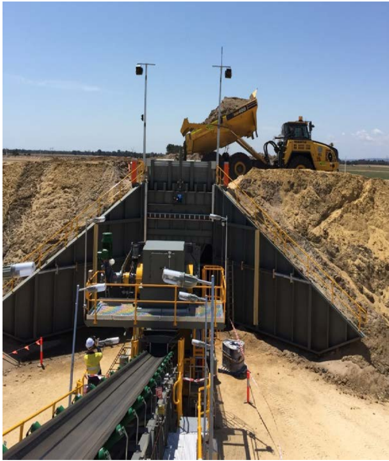
Figure 1: First truck unloading ore into the MFU at Keysbrook
