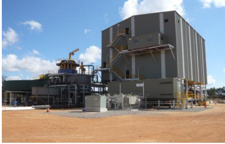
Figure 1: Keysbrook Wet Concentrator Plant (WCP)
