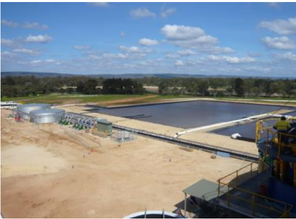
Figure 2: Process water dam and pumps at Keysbrook
