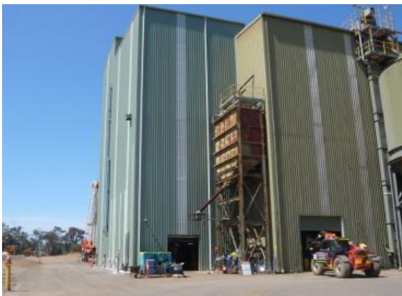
Figure 4: Completed Annexe at Picton Mineral Separation Plant (MSP)
