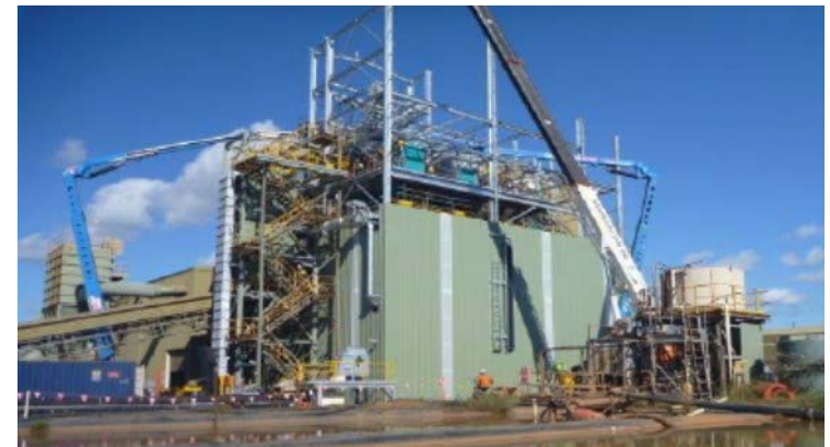
Steel erection at Picton MSP
