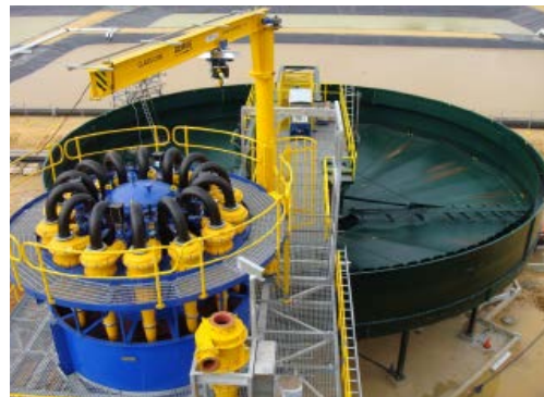
Figure 4: Thickener awaiting sealing
