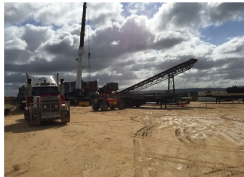
Figure 5: MFU assembly in progress
