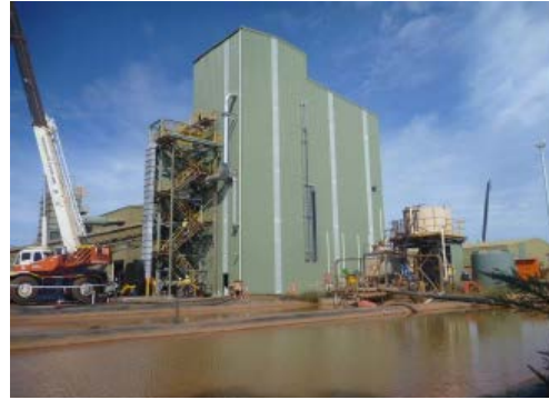
Figure 3: Annex construction at Picton
