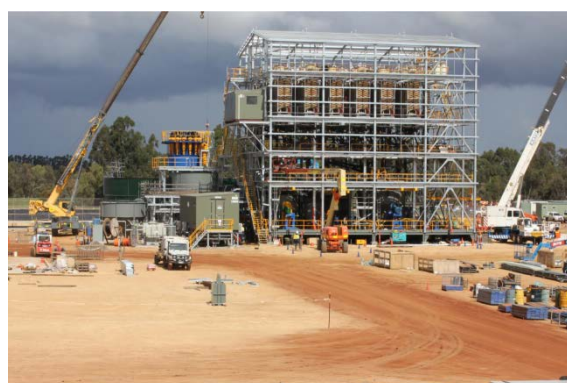
Figure 3: Wet Concentrator Plant (WCP) under construction
