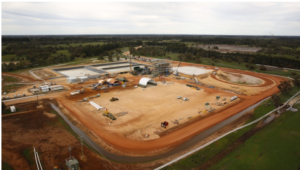
Figure 1: Keysbrook mine site construction activities
