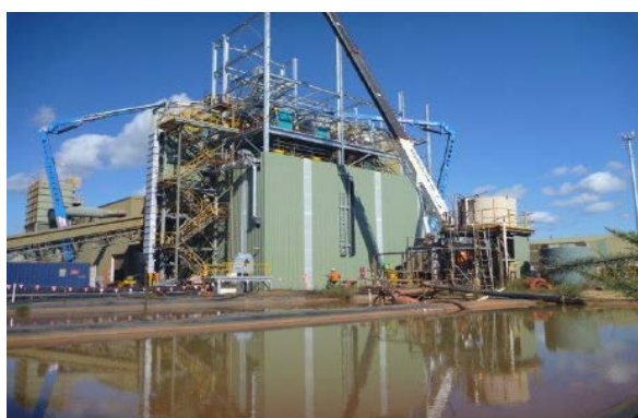
Figure 2: Construction activities at the Picton Mineral Separation Plant
