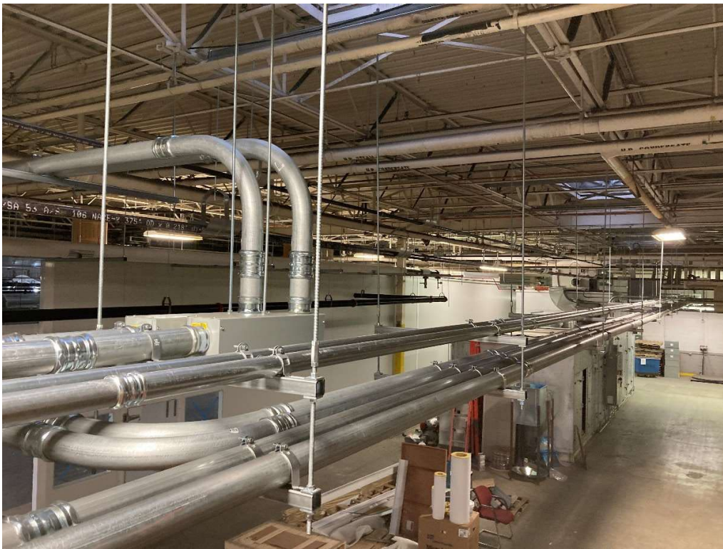
Figure 3: Low Bay electrical conduit installation
