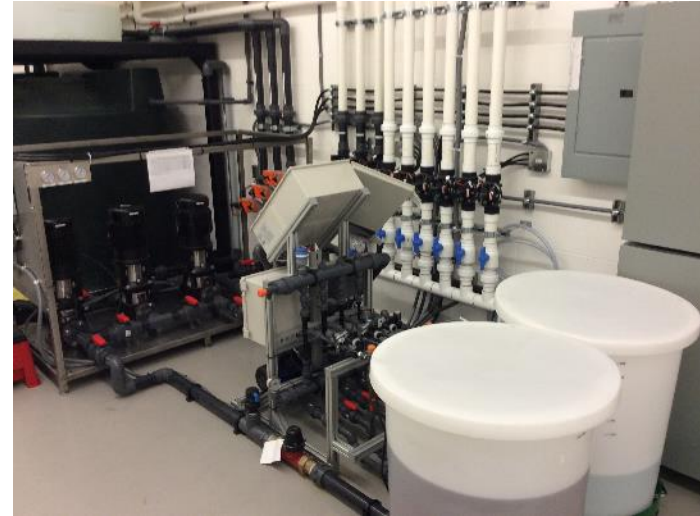
Figure 2: Duncan Facility automated fertilizer system.
