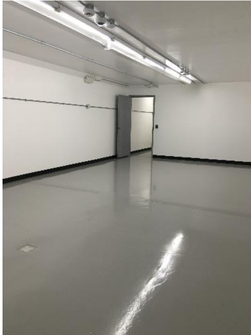
Inside the Vault
