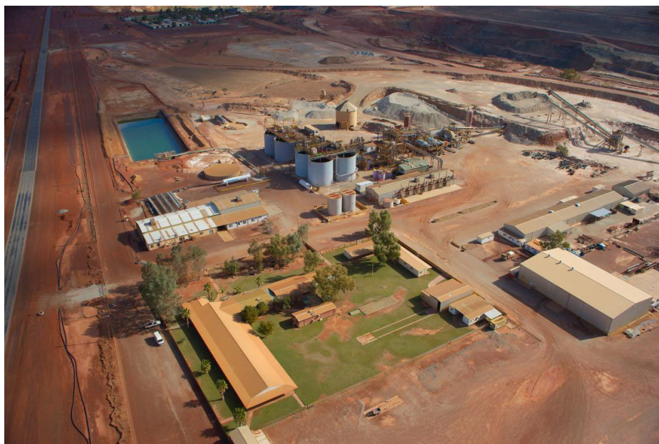
[ Picture: The 2.5 Mtpa Bluebird plant and associated infrastructure ]
