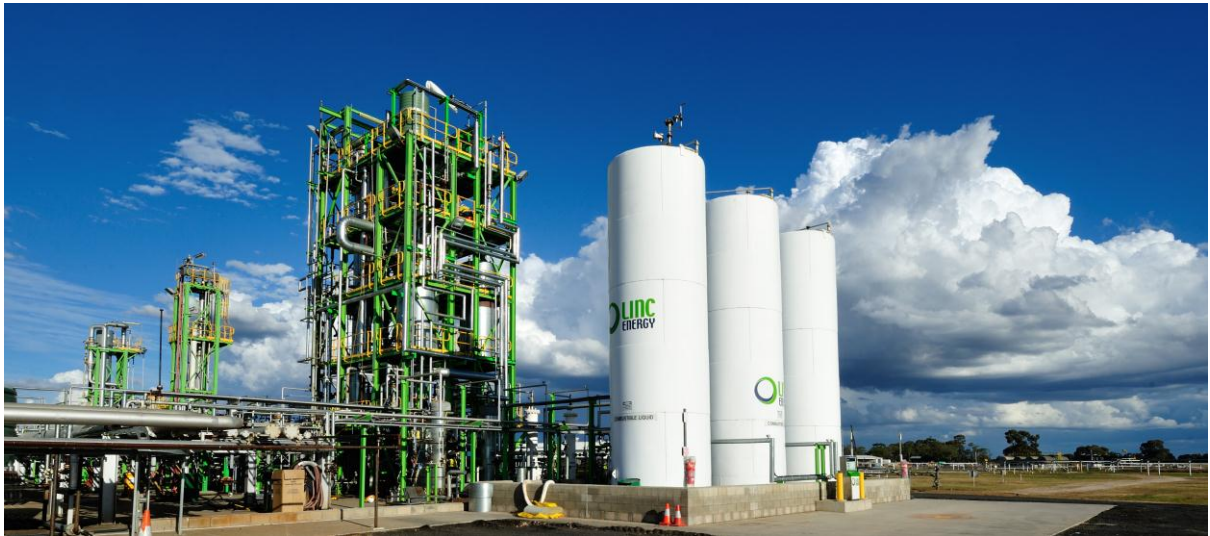
Linc Energy's GTL Facility
