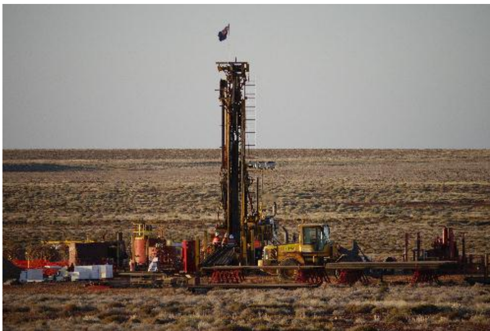
Above: Linc Energy's Wirrangulla Hill 1 drill site on PEL 122, South Australia.
