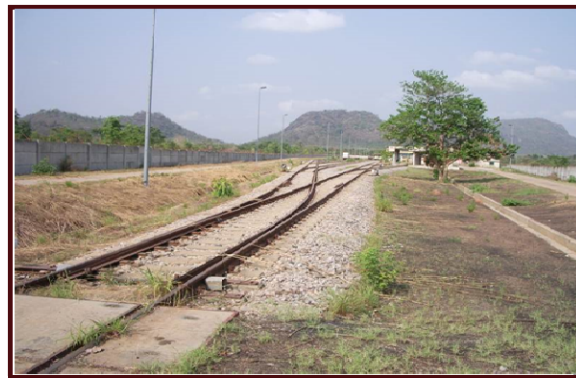
Existing Itakpe/Ajaokuta Railway
