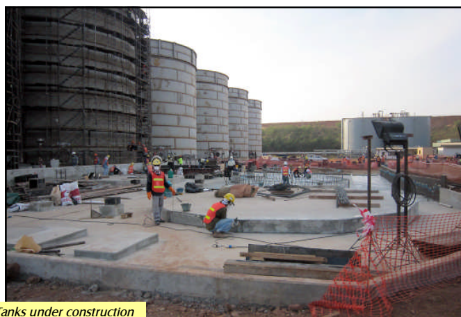
Grinding Plant and Elution Tanks under construction
