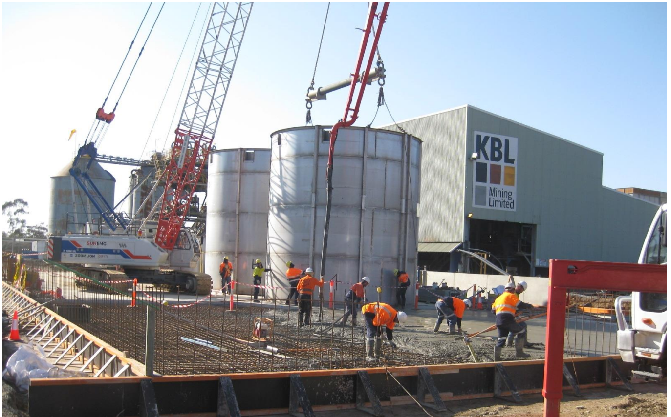
Photograph 2. CIL construction (July)
