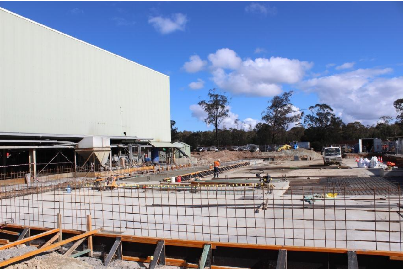
CIL plant foundations
