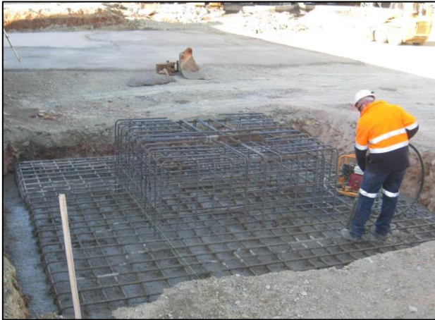
Photos 3 and 4. CIL Plant – Tower crane foundations
