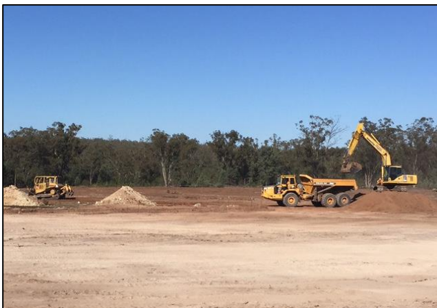
Photo 1. Topsoil stripping at Pearse
