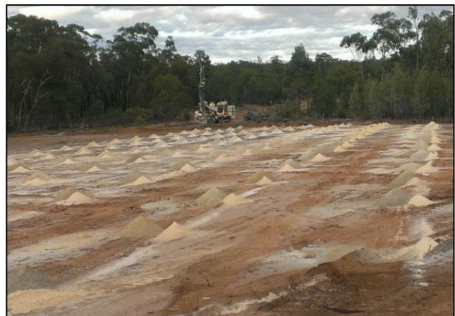
Photo 2. First blast hole pattern for Pearse Open Cut
