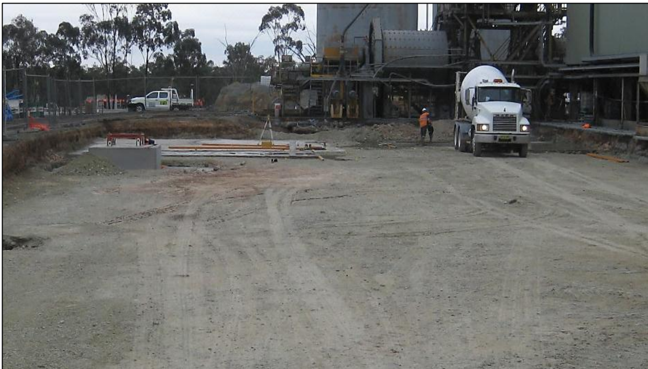
Photo 5. CIL Plant – Concrete foundations
