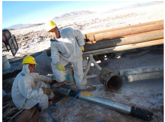
Installing pump at production bore field
