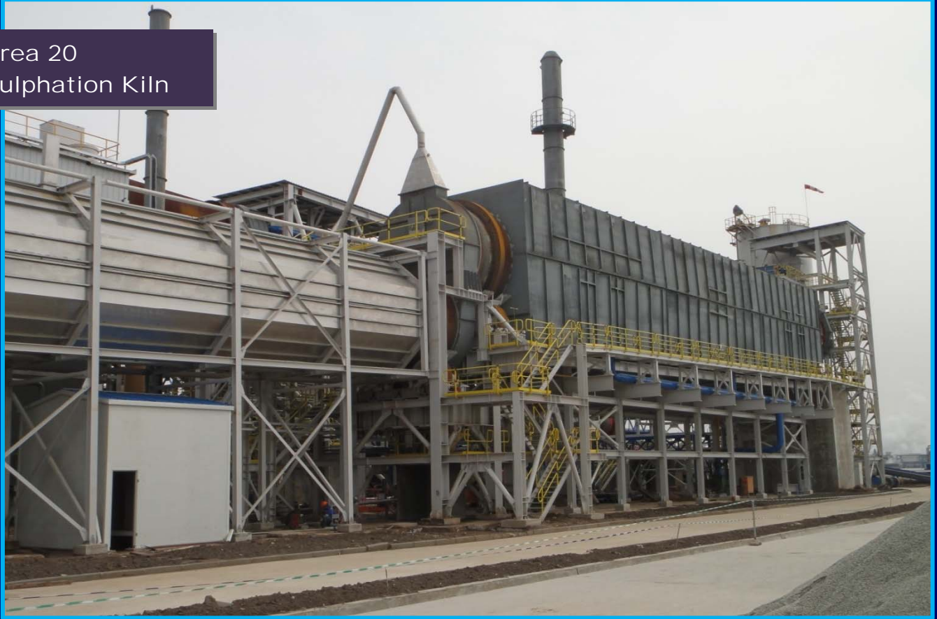
Sulphation kiln and cooler ready to accept beta spodumene
