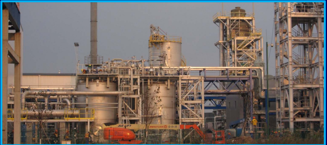
Purification crystalliser and digester tanks
