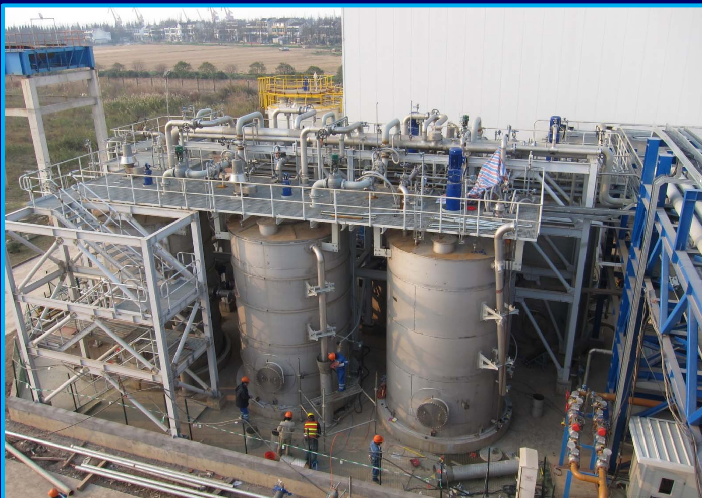
Digester tanks at purification plant
