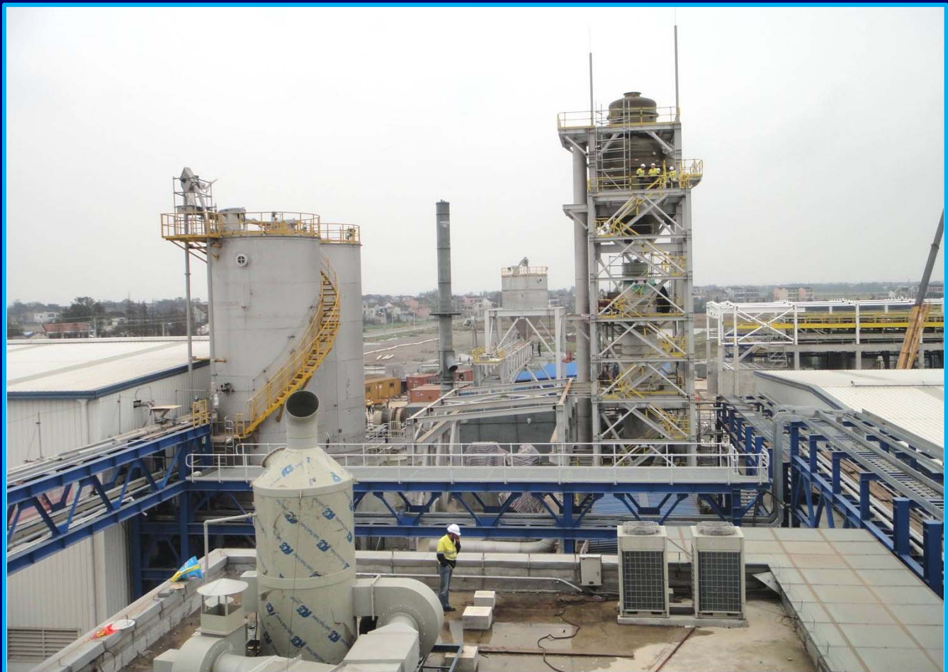
Final product bins and sodium sulphate crystalliser
