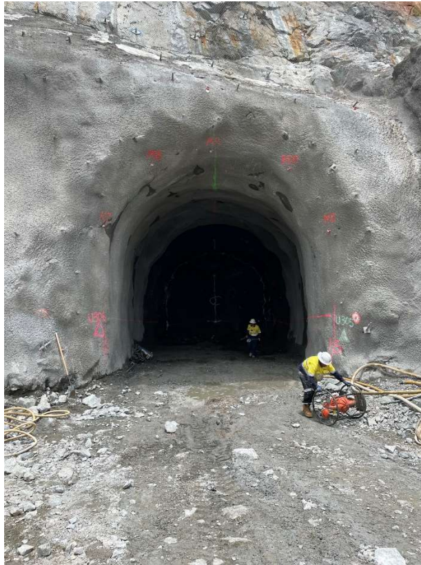
Figure 3: MAT following muck out and descaling operations
