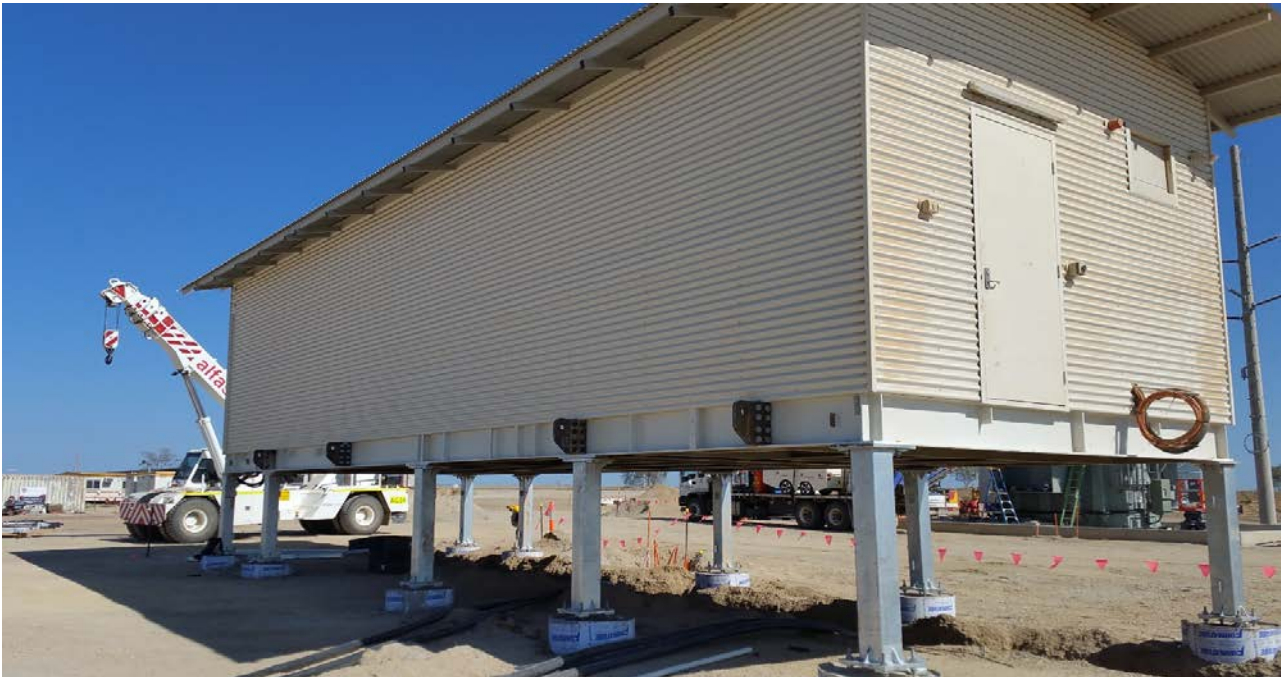
Figure 3: Installation of control room.
