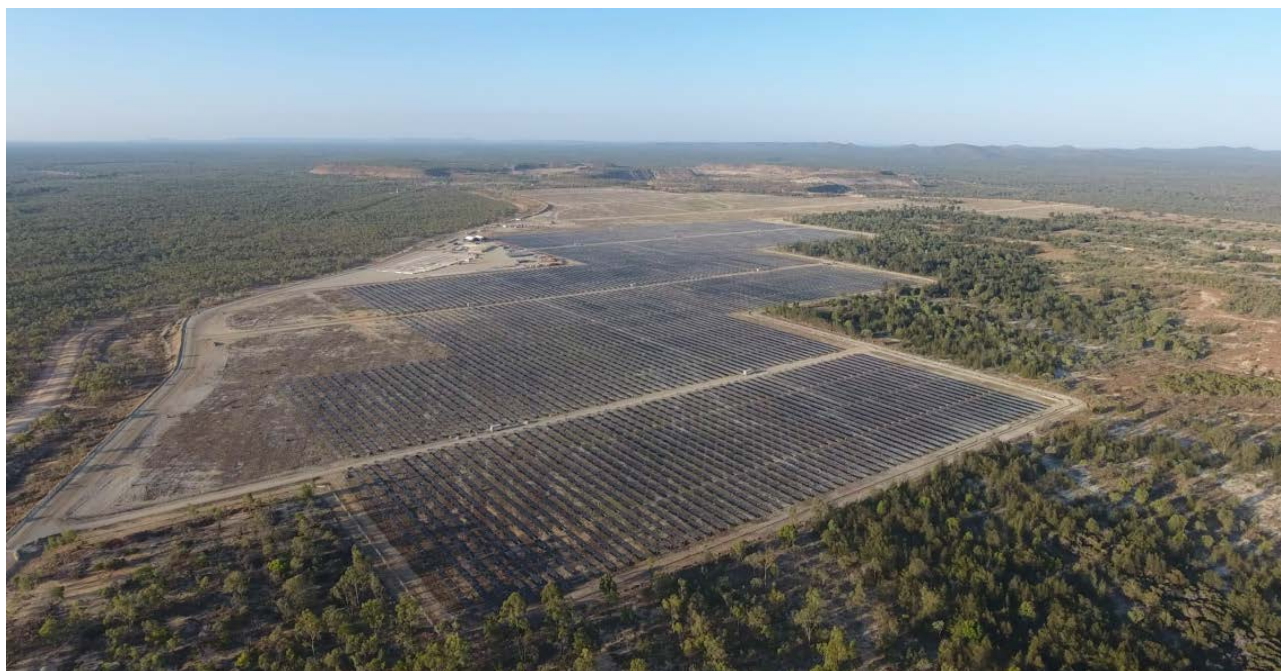
Figure 1: Aerial view of a section of the 50MW Kidston Solar Project.
