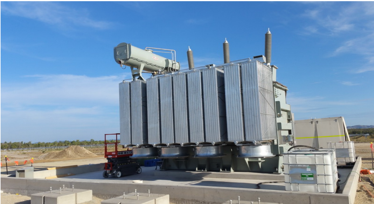
Figure 2: Installation of transformer.
