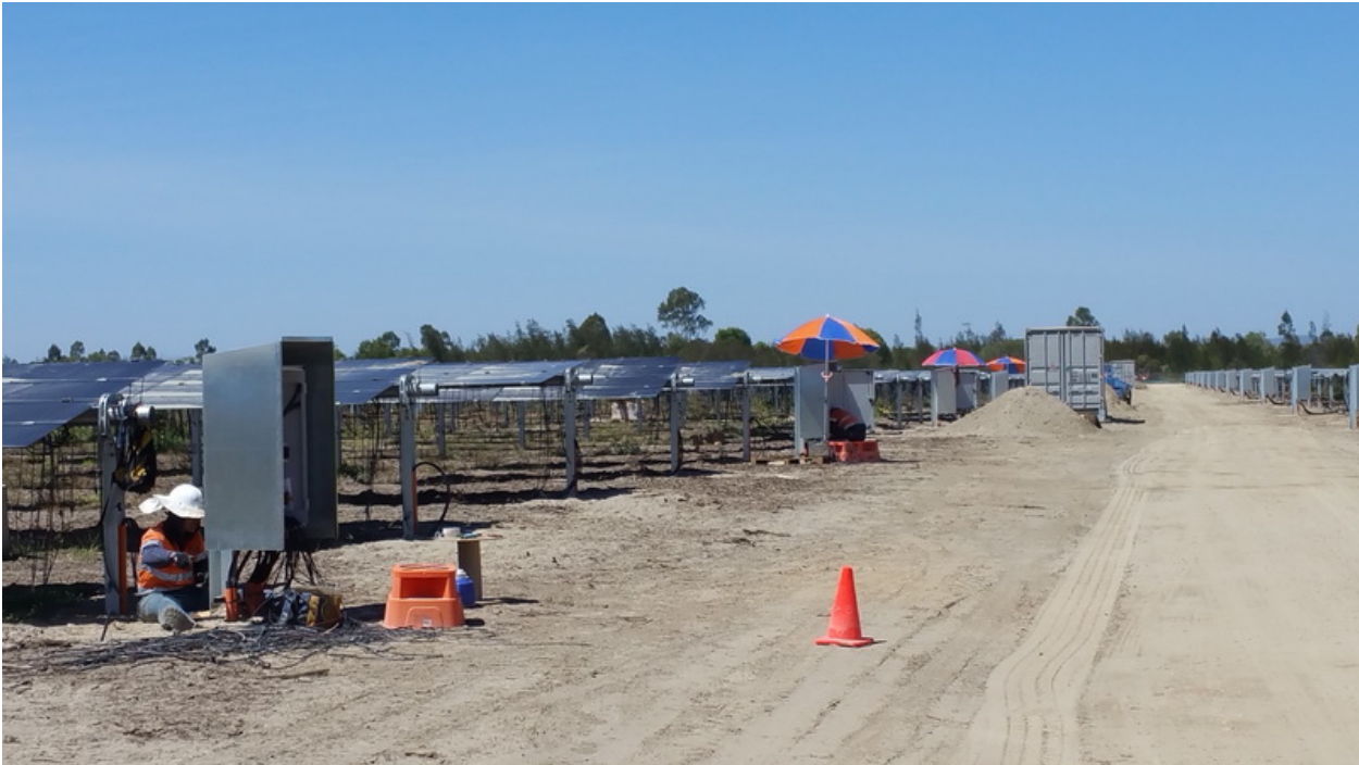
Figure 5: Electrical technicians terminating cables at the combiner boxes.
