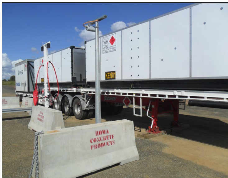
Figure 5: Loading post and virtual pipeline trailers.
