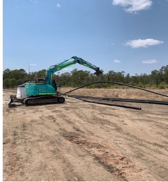
Figure 2: Installation of gathering system
