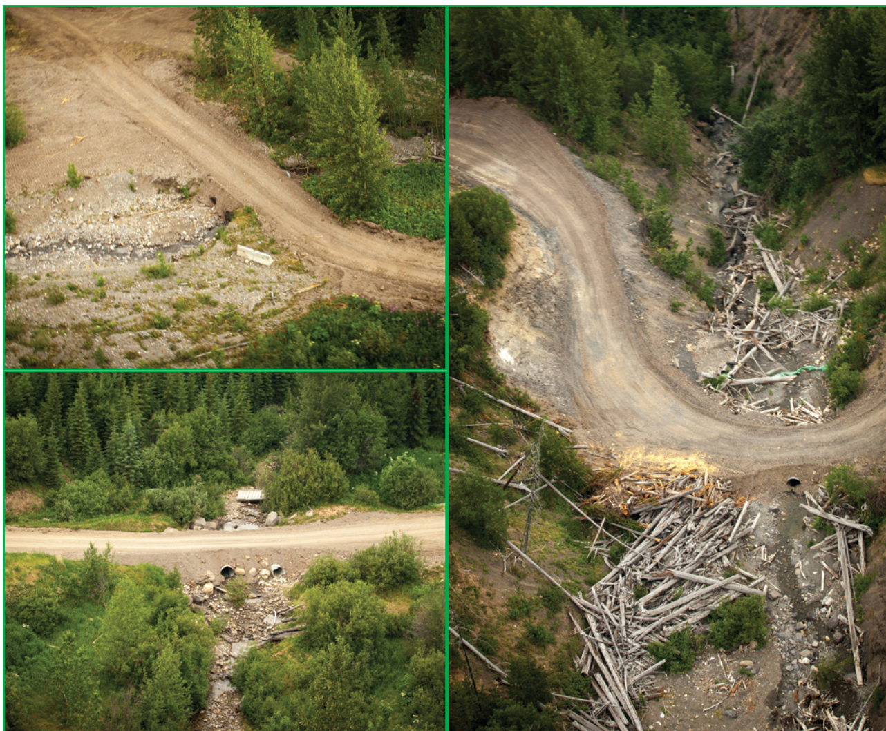
Figure 2 — Road improvements at Wapiti – installation of culverts across creeks
