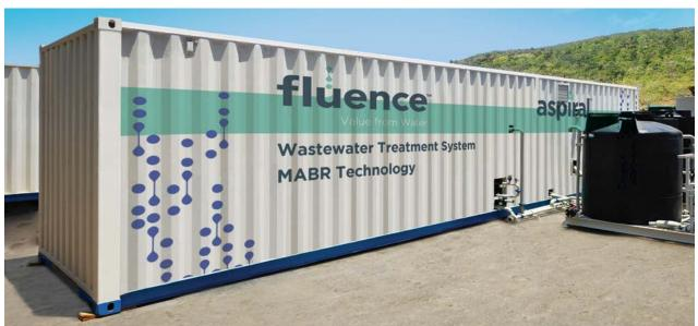
Aspiral<sup>™</sup> was chosen for this project in part due to its small footprint and ability to reliably achieve Class 1A effluent.
