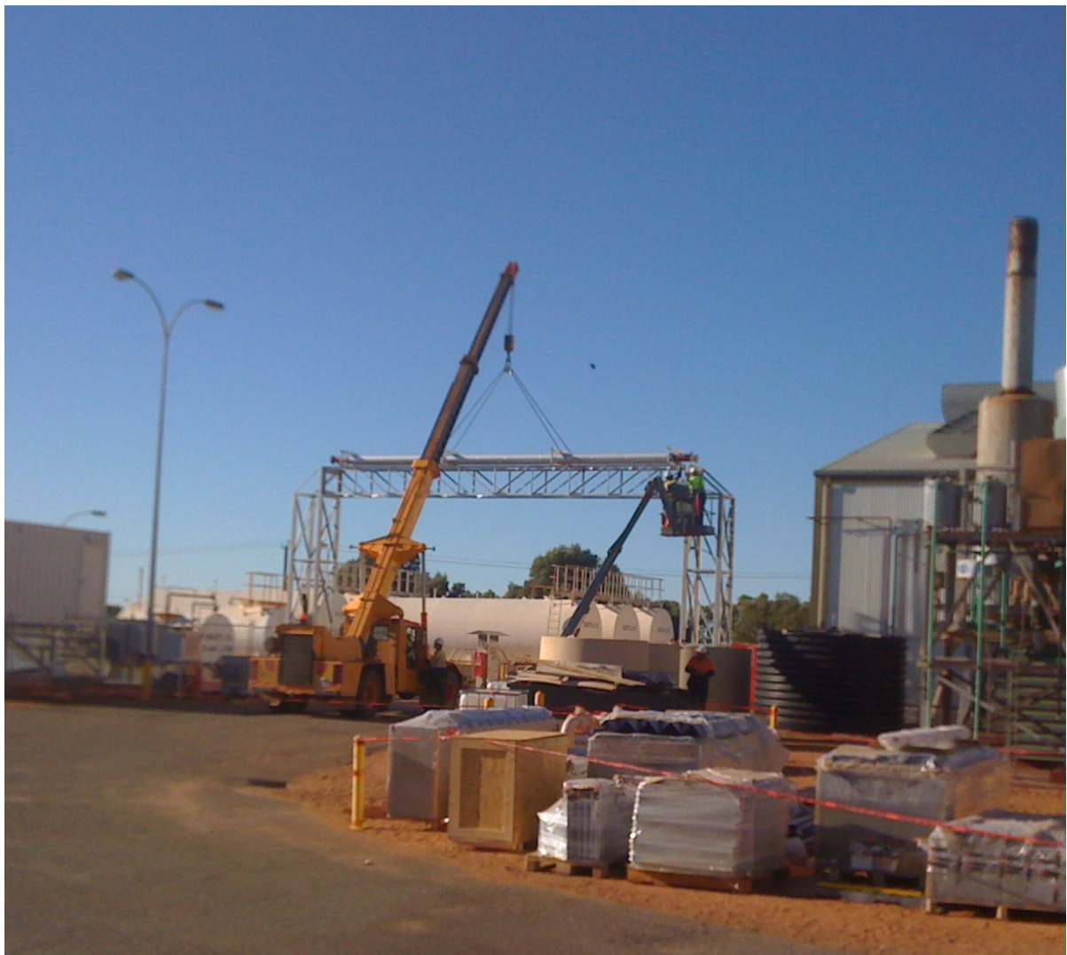
Figure 1 – The pipe bridge being lowered into place
