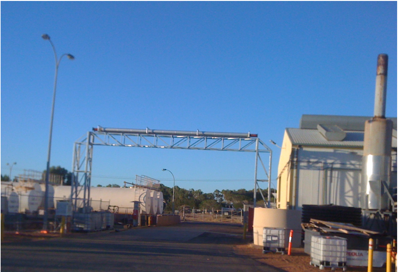
Figure 2 – The completed pipe bridge
