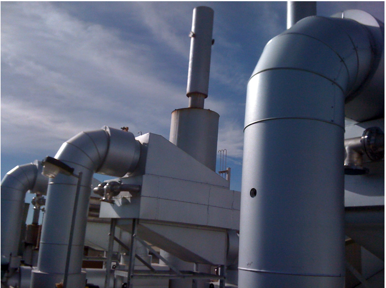
All three heat recovery units installed in Carnarvon
