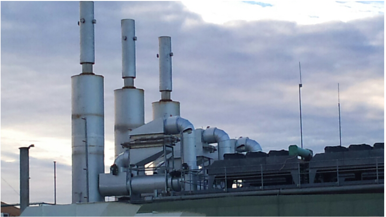
All three heat recovery units installed in Carnarvon
