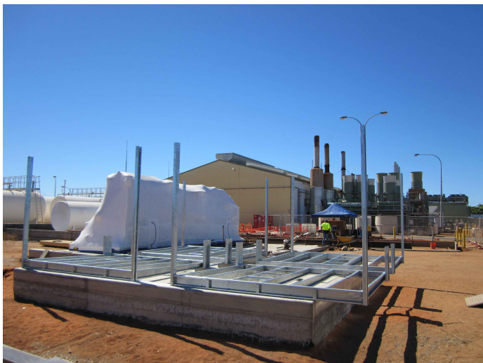
Enerji's Opcon Powerbox – installed on site in Carnarvon with the cooling tower assembly occurring in the foreground
