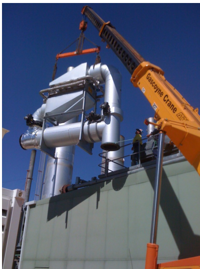
Enerji's first heat recovery unit being installed at Carnarvon
