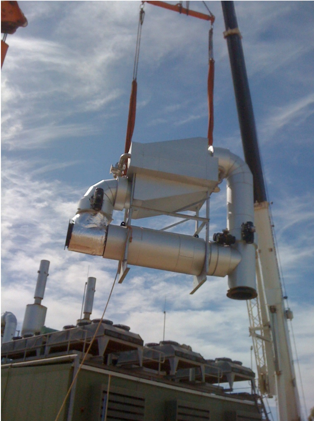
Figure 1–The second heat recovery unit (HRU) is installed in Carnarvon
