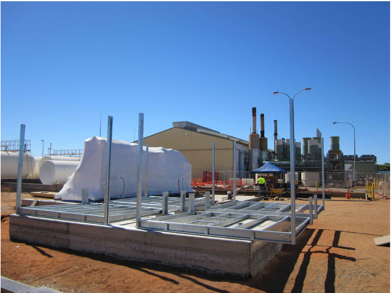
Figure 1–The cooling tower being assembled alongside the Opcon Powerbox in Carnarvon
