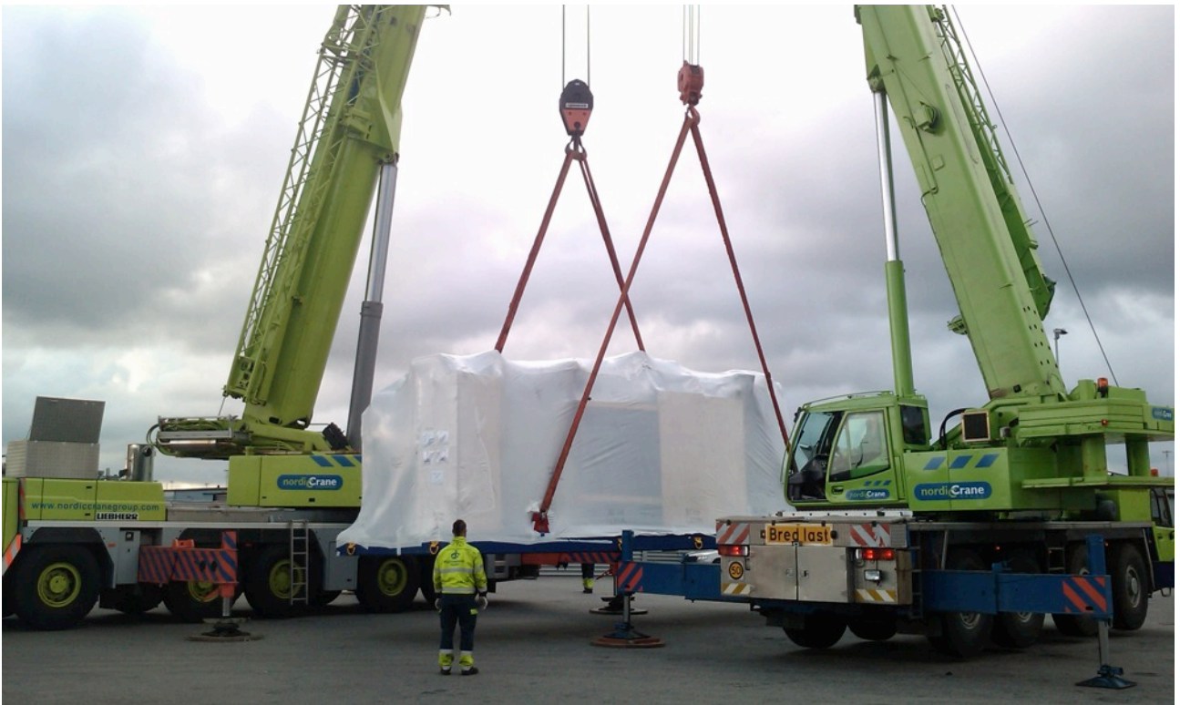
Figure 5 - Unloaded and ready to transfer
