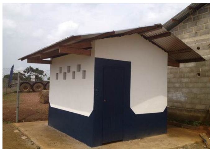
Figure 14: New Ablution Facilities at the Mayoko School
