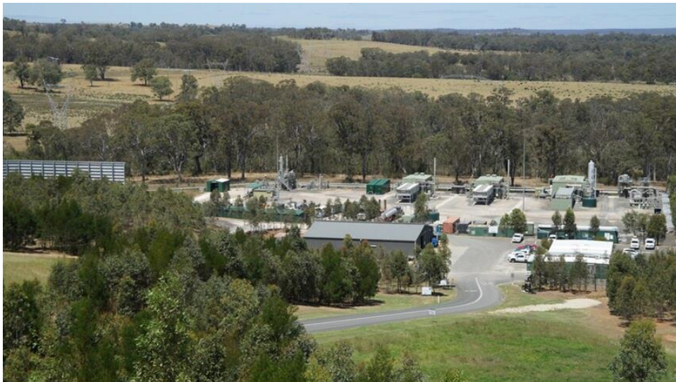
Rosalind Park Gas Plant, Menangle, New South Wales
