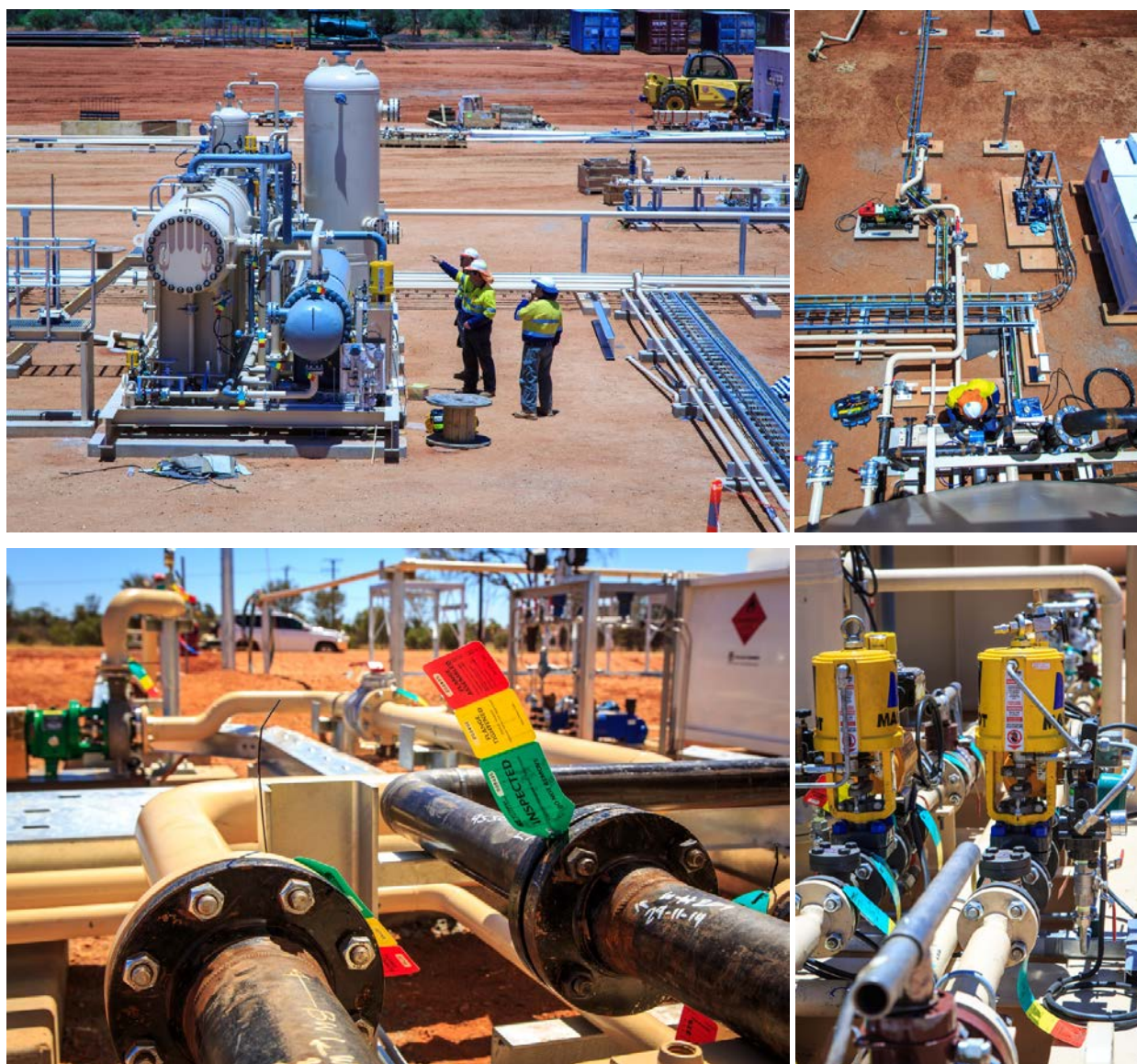
Figure 3: Commissioning underway on Dingo Project
