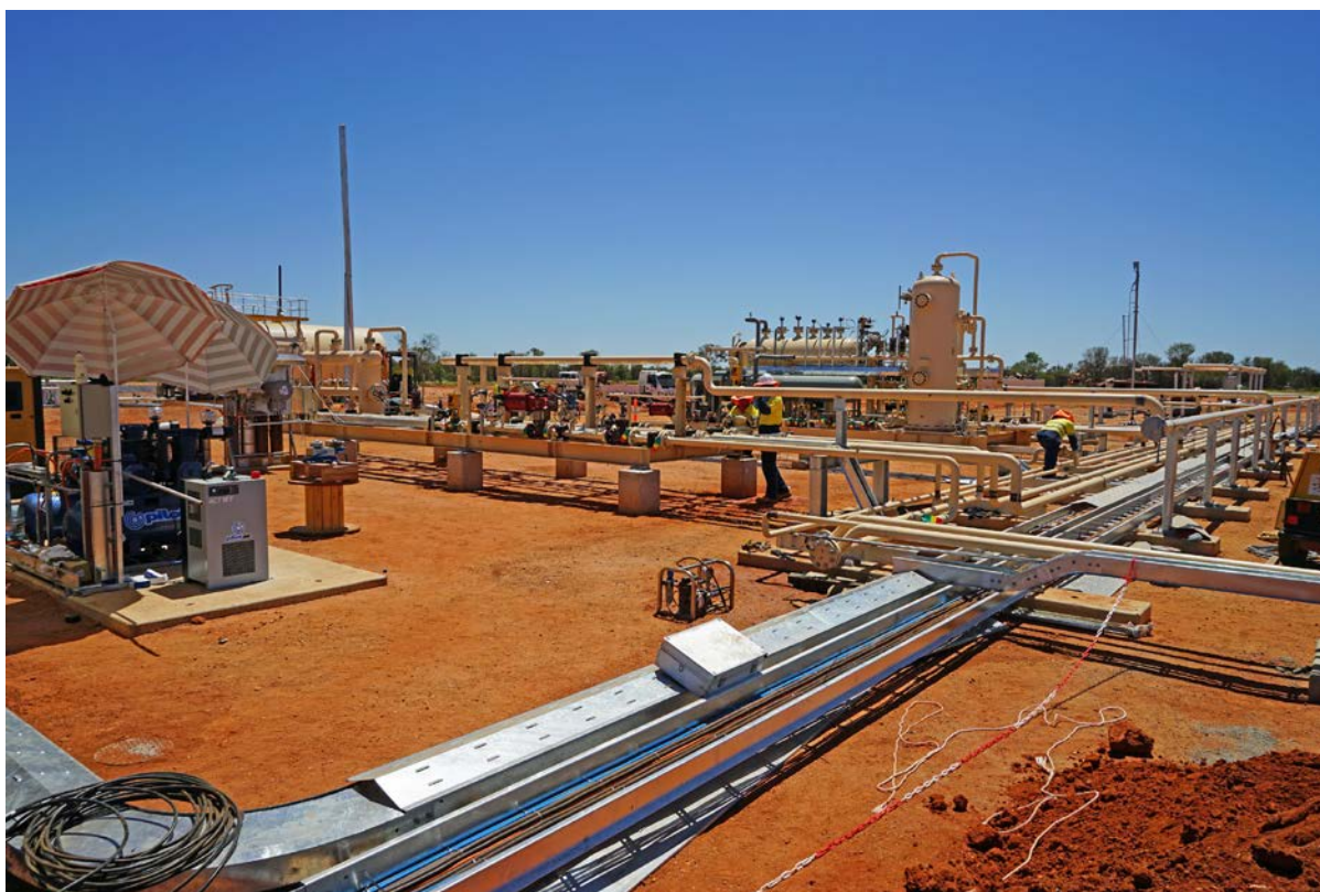
Figure 2: Brewer Estate Gas Plant (Dingo Project) showing good progress in mid-February
