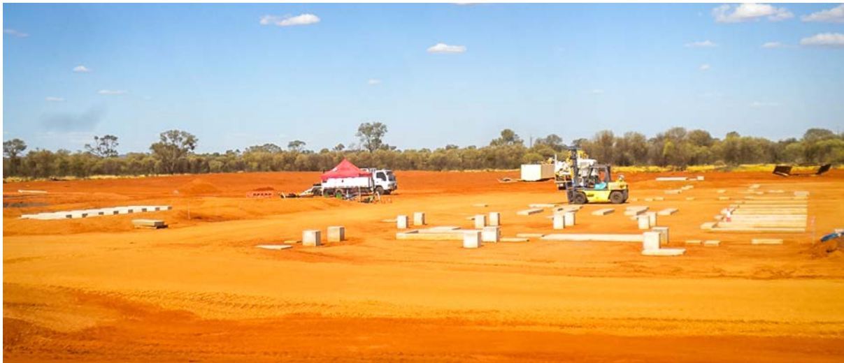
Figure 8: Footings at Brewer Estate ready to receive prefabricated gas plant modules
