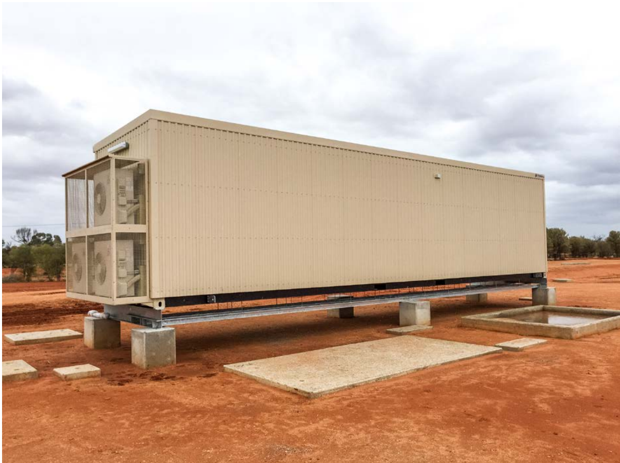
Figure 5: Electric Control Room; prefabricated and delivered to site
