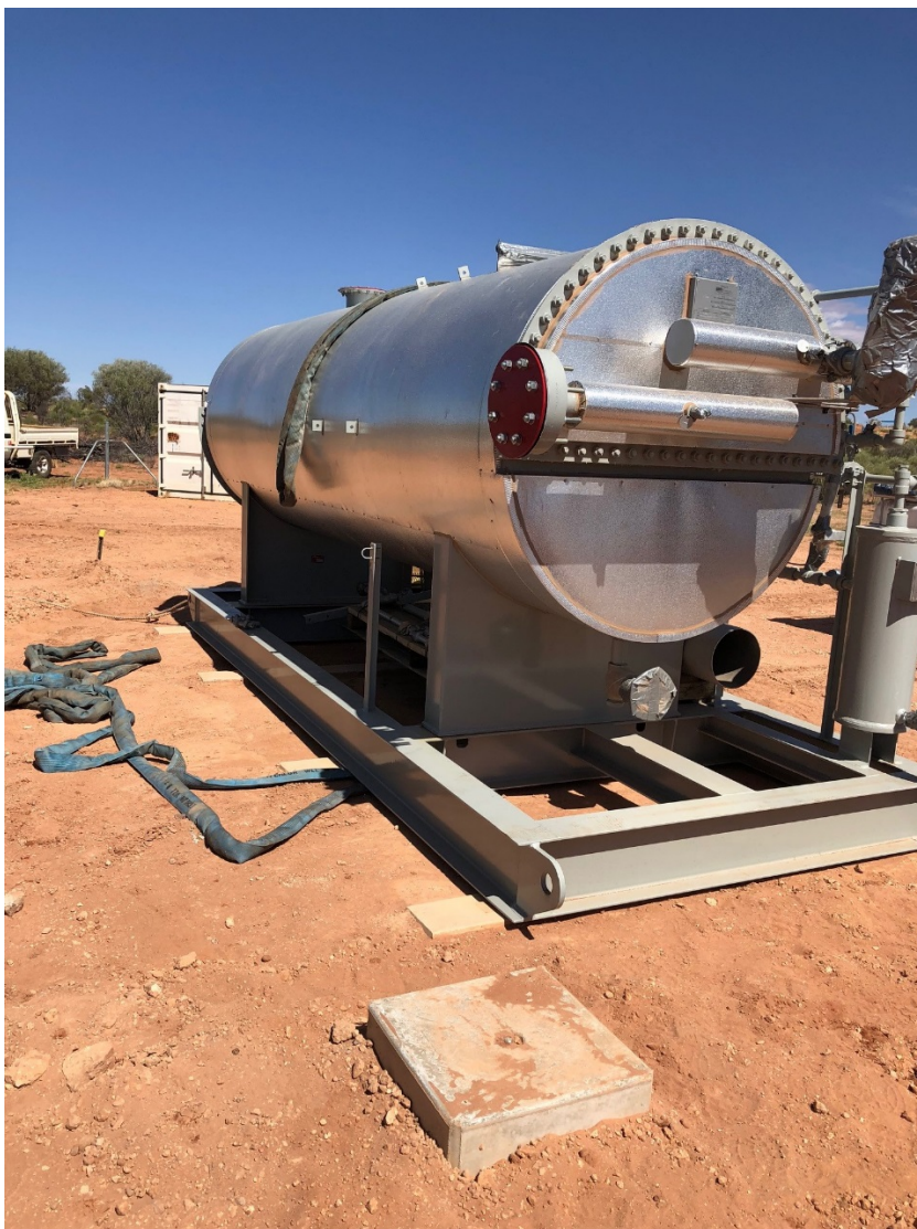
Figure 2: Water bath heater for Dingo situated on-site.
