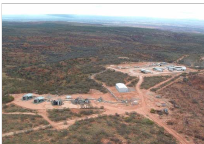
Palm Valley Gas Plant Facilities
